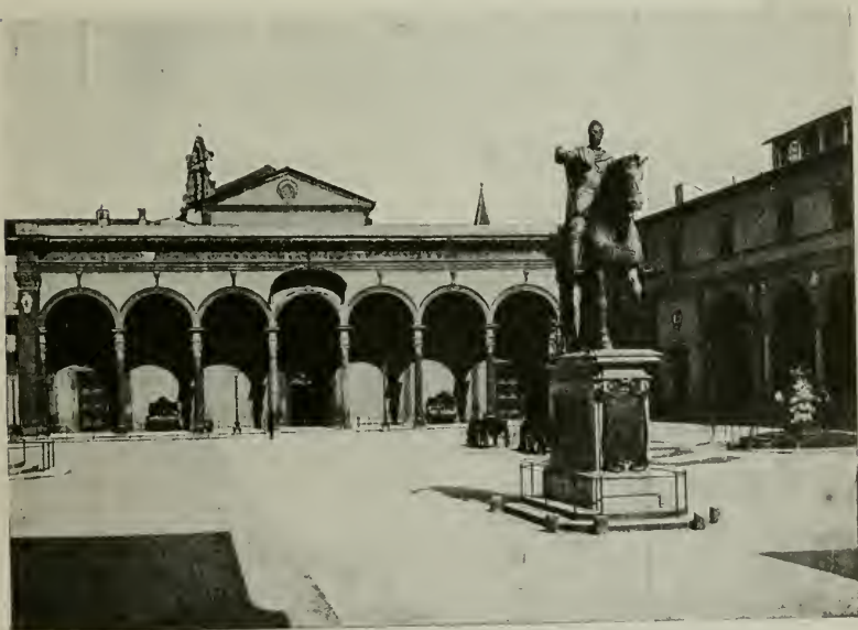
LOGGIA OF THE CHURCH OF SS. ANNUNZIATA, FLORENCE. Antonio 'a Sangallo an' G. B. Cacciari, Archts.
